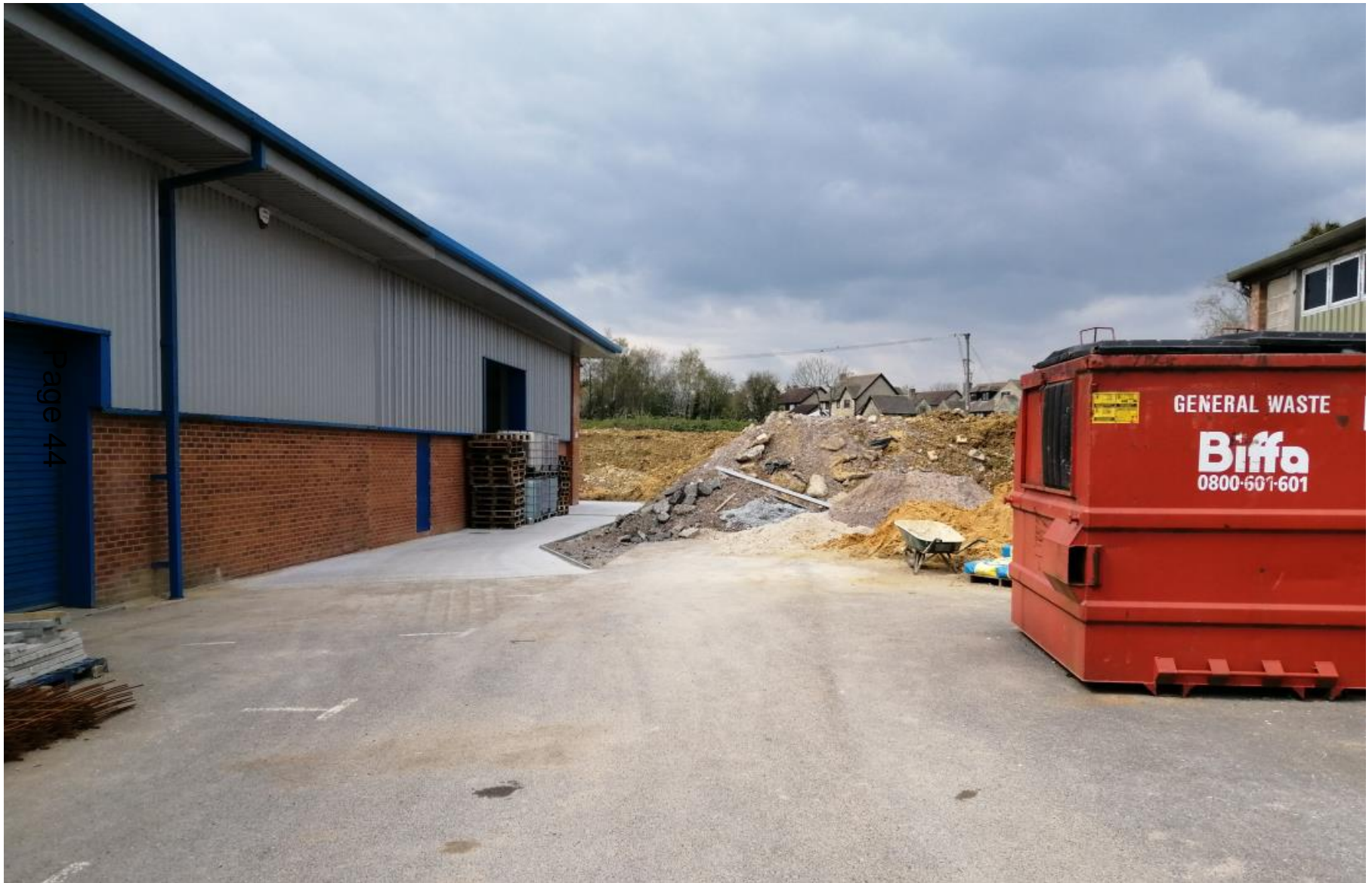
View of the extended unit 8 permitted under application 19/06790/FUL
