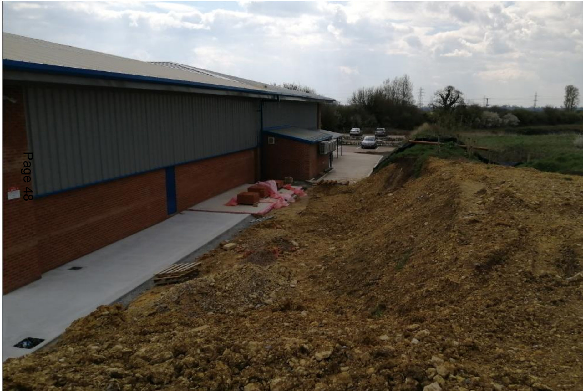
View from top of bund looking south to unit 9
