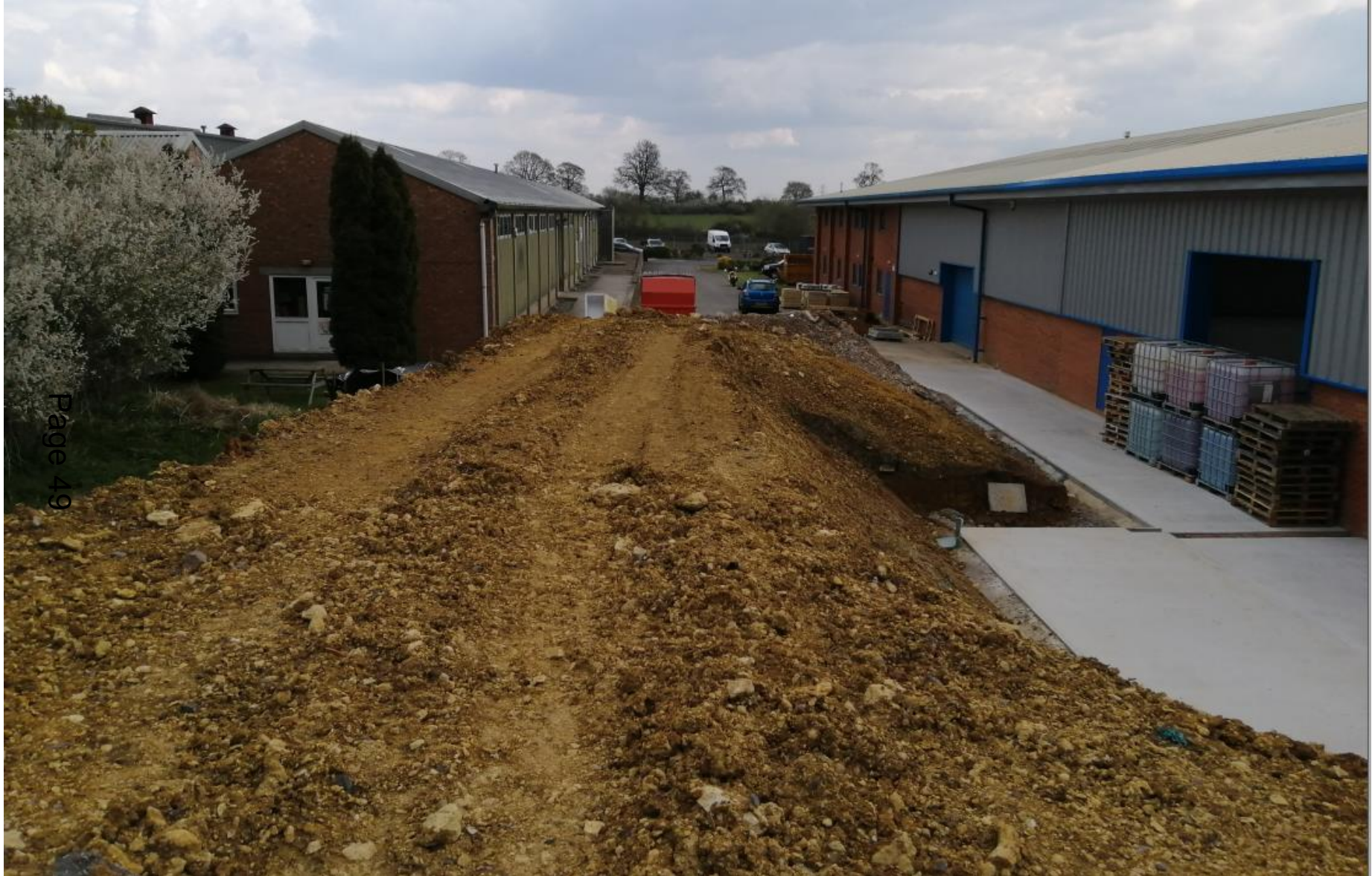
View from top of bund looking east down service road
